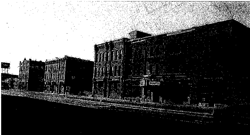
South side of Washington Avenue, west of 10 th Avenue, view looking southeast. Mead & Hunt photograph.
