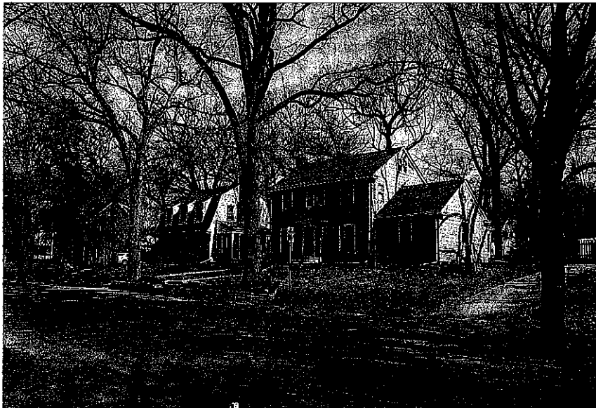
North side of East River Terrace, east end of block, view facing northwest. Mead & Hunt photograph.
